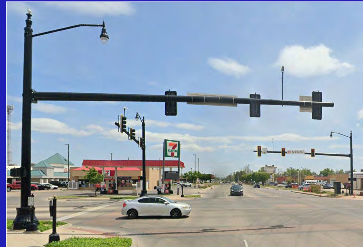
Decorative Poles @ NW 50 th & MacArthur Intersection
